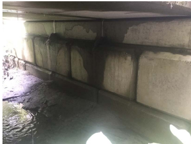
Left Bank Abutment when facing downstream
