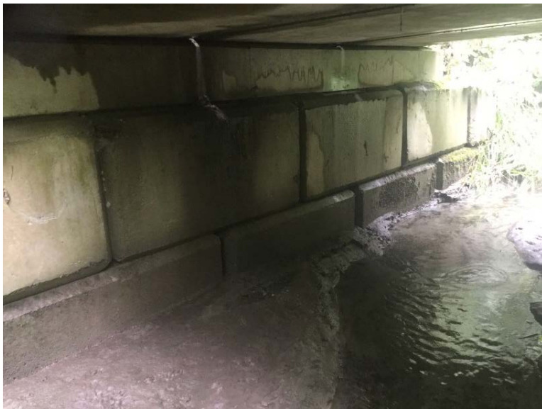
Right Bank Abutment when facing downstream
